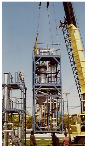
900 lb/hr. Isopropyl Acetate/Isopropanol package distillation system, 316 SS with automatic stripping and process heat recovery.
