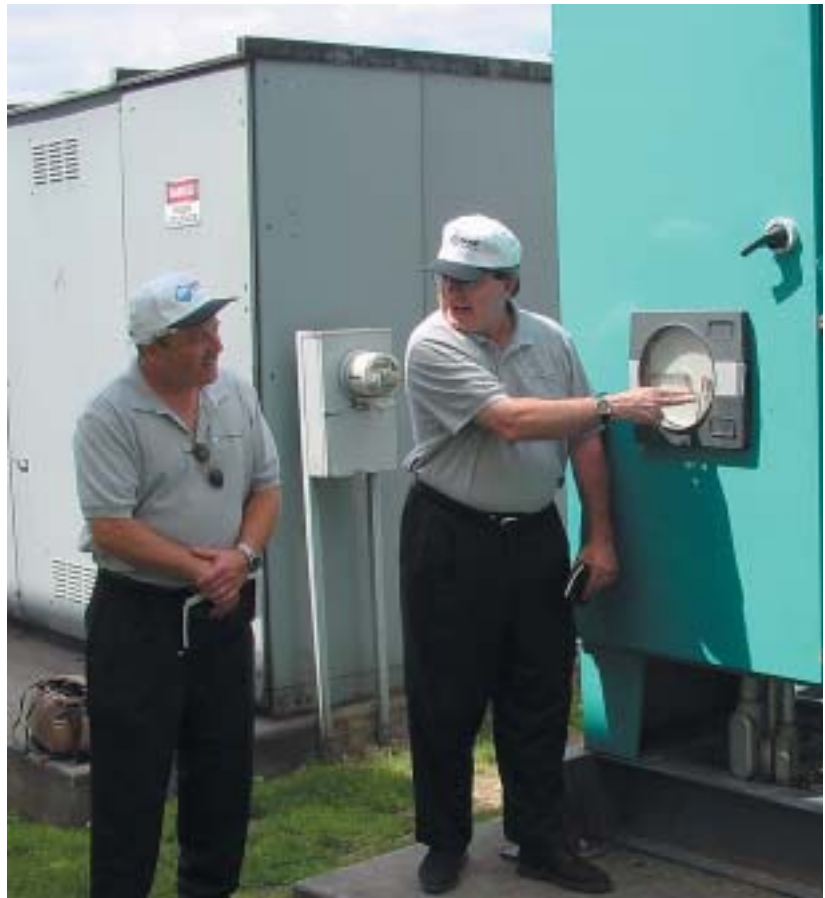
CSM's Complete Compliance Program includes on-site engineering throughout the project.
