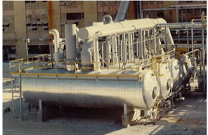
80,000 CFM ADSOLV Acetone Recovery System - for Synthetic Resin
